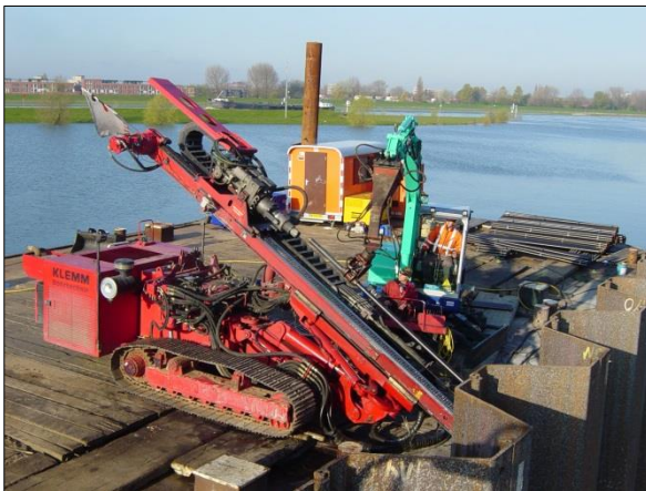
Figure 20. Crawler rig, tieback installation
