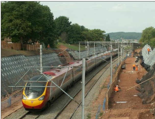
Figure 1. Hollow bar soil nails
