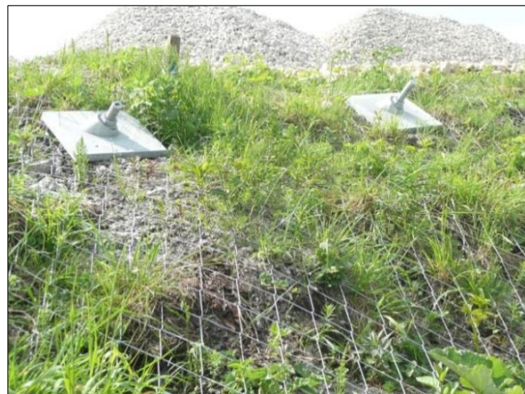
Figure 6. Articulating wedge boss
