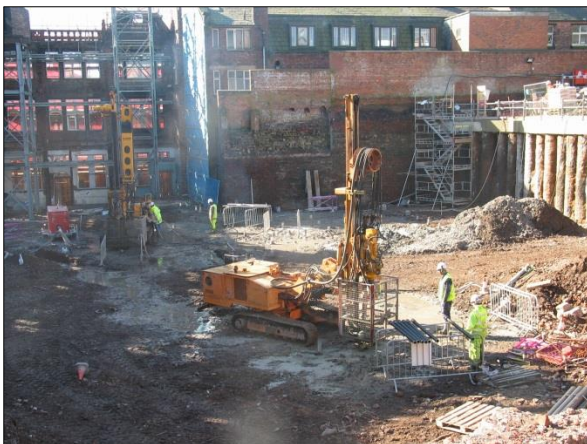
Figure 7. Installation of hollow bar micropiles. Figure 8. External sleeve on micropiles
