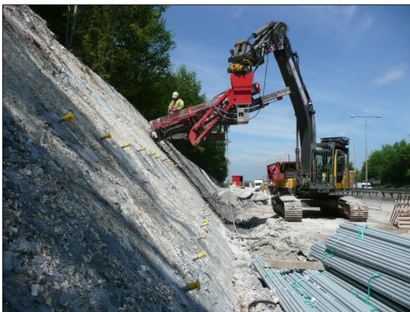
Figure 16. Excavator mounted drill boom Figure 17. Long reach excavator drilling
