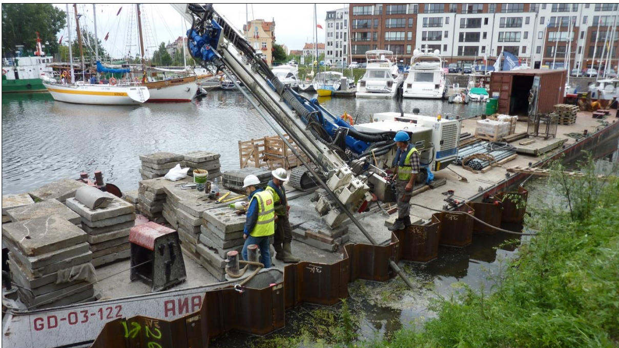
Figure 9. Hollow bar tension piles for sheet pile tieback
