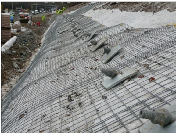
Figure 5. Lipping of bearing plates
