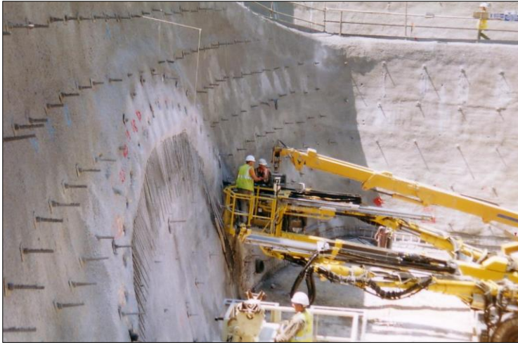
Figure 18. Portal rock bolts installed with boomer
