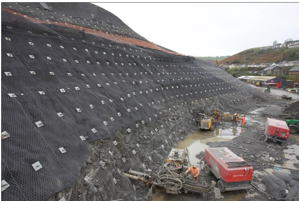
Figure 3. Hollow bar soil nails with top bar galvanizing, for slope stabilisation
